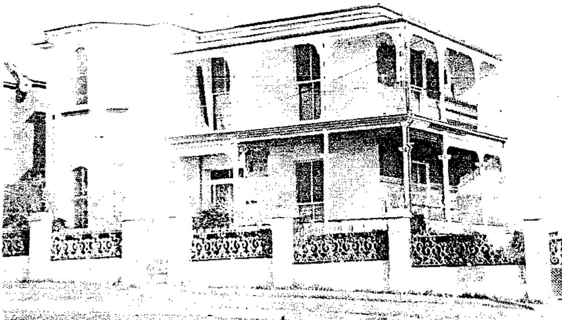
FIGURE 70: 'Clandulla,' No.144 Cowper Street. Recent removal of stucco revealed the neat, smooth stonework used in the house's construction.
